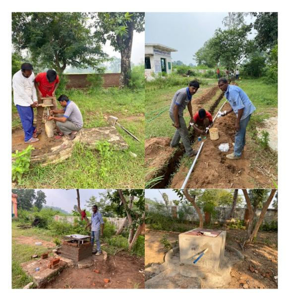
4. An armoured 4-core underground electric cable was installed providing secure and safe electric supply from the transformer to the school. All classrooms have electricity. 2 fans have been installed in each of the larger classrooms and 1 each in the 2 smaller rooms. Each room has 2 light points and 5 power points. All power supply lines are underground.
